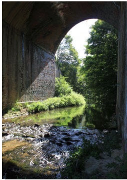
River Witham below the existing rail viaduct
