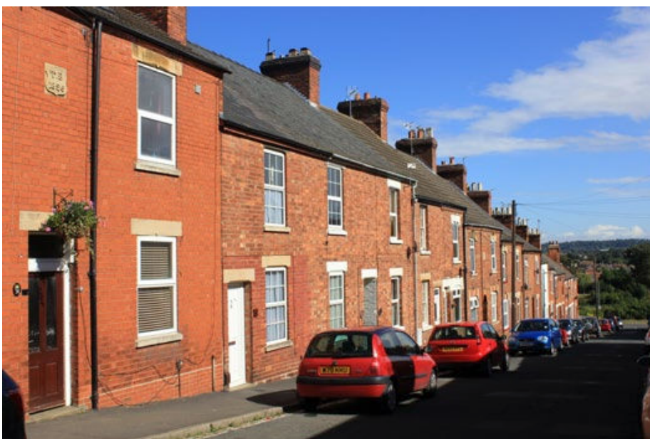
Existing street on the sloping landform surrounding the town
