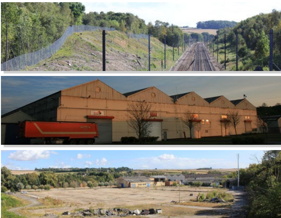
Rail corridor and industrial works in the north west of the site
