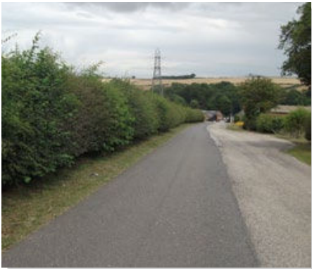
Access road to existing water treatment works
