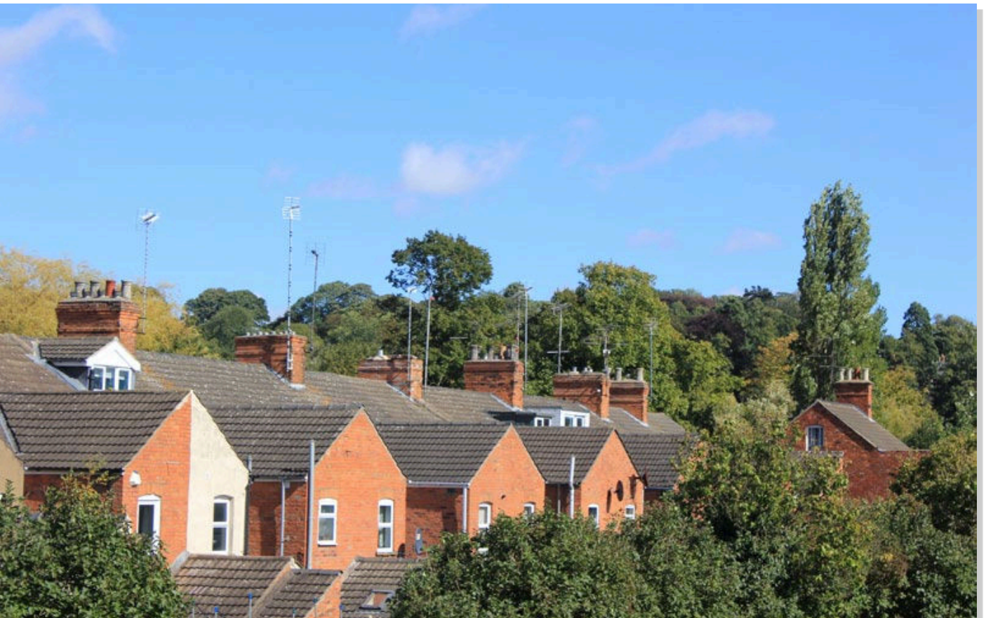
Existing properties close to the River Witham
