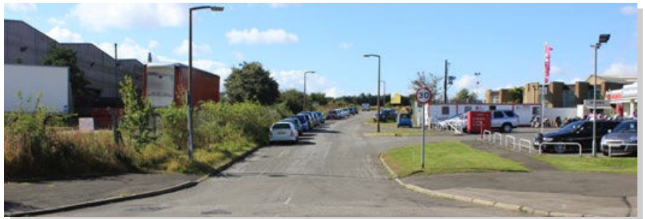
The future link road to the A1 will extend to the west of the B1174
